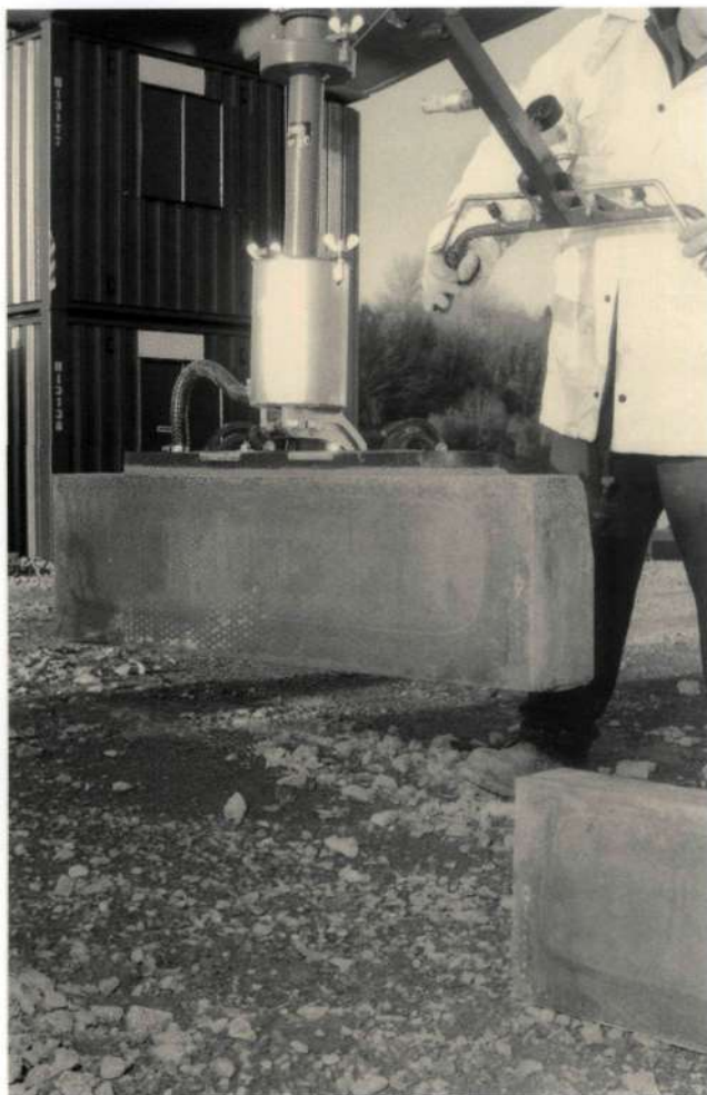
Figure 38 Handling kerbs using a vacuum lifter
