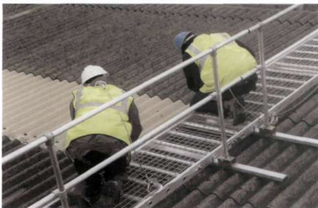
Figure 27 Workmen wearing harnesses attached to a work positioning line, which is fitted to the staging
