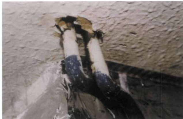
Figure 48g Painted asbestos-containing textured coating on a ceiling
