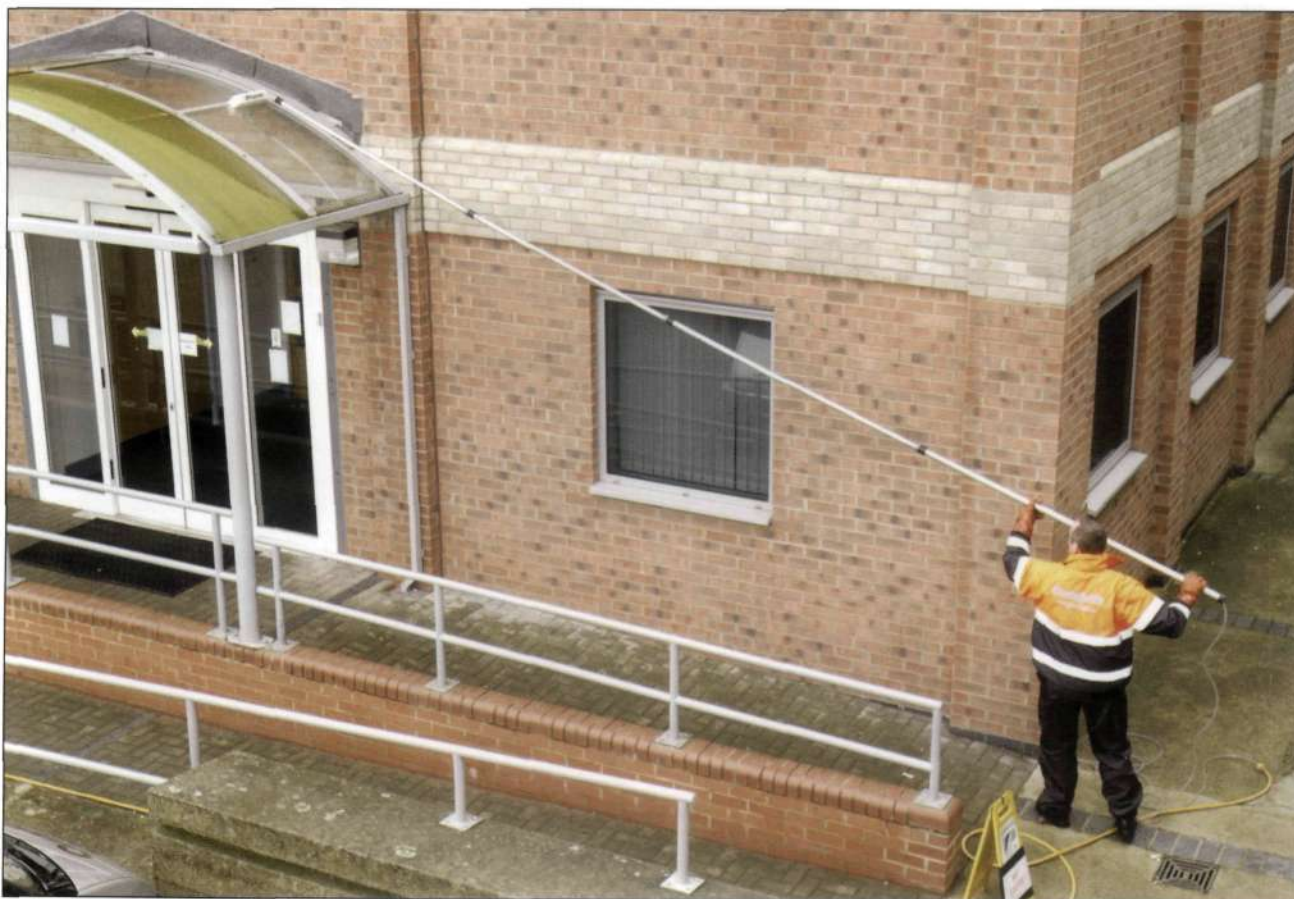
Figure 8 Using a long pole to avoid working at height
