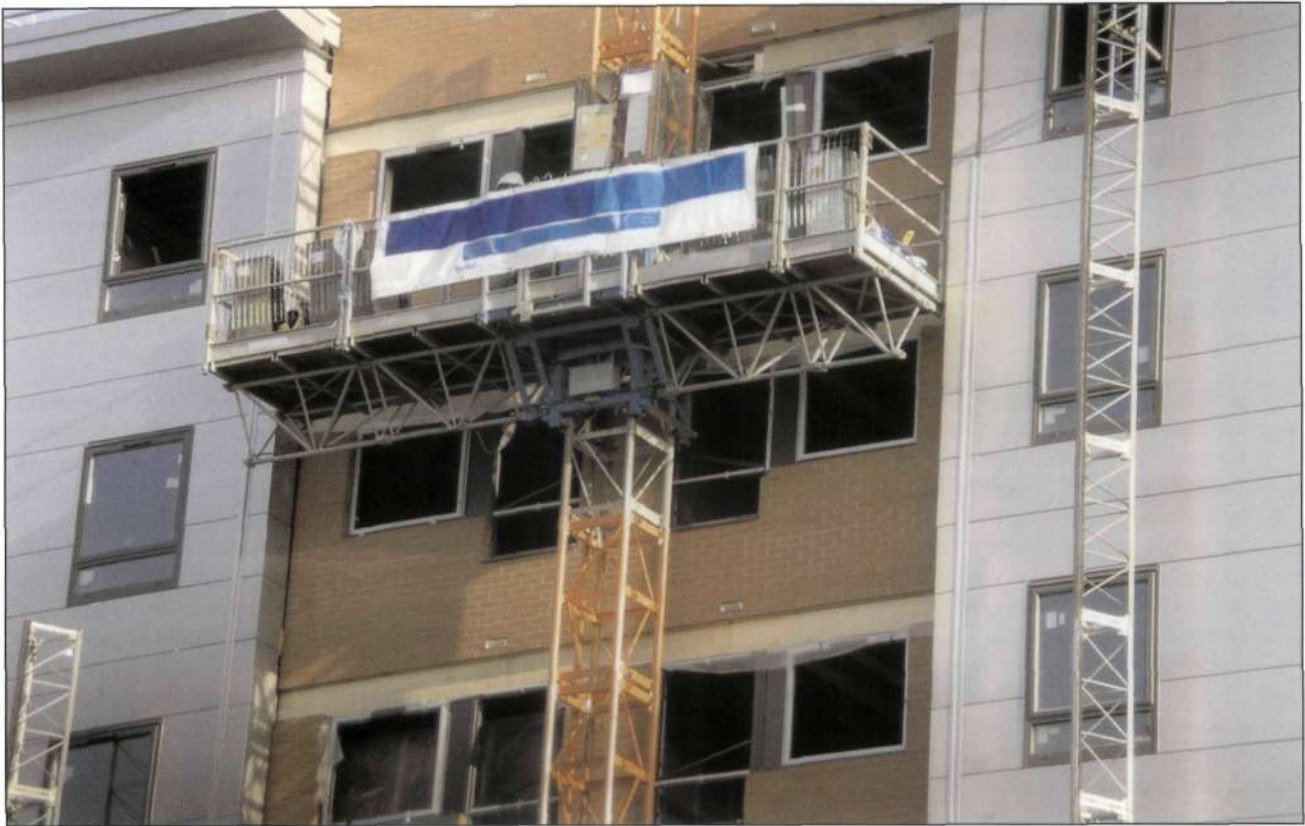
Figure 14 A mast climbing work platform
