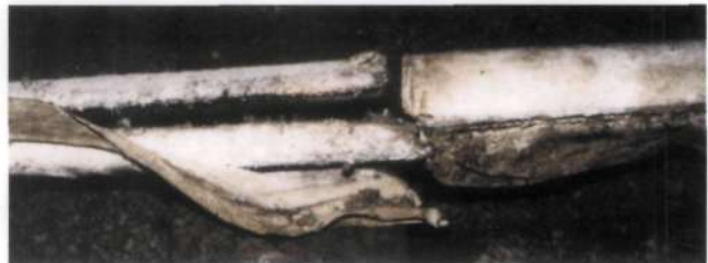
Figure 48a Asbestos-insulated water pipes showing evidence of maintenance work damage, with detached preformed sections and calico wrapping
