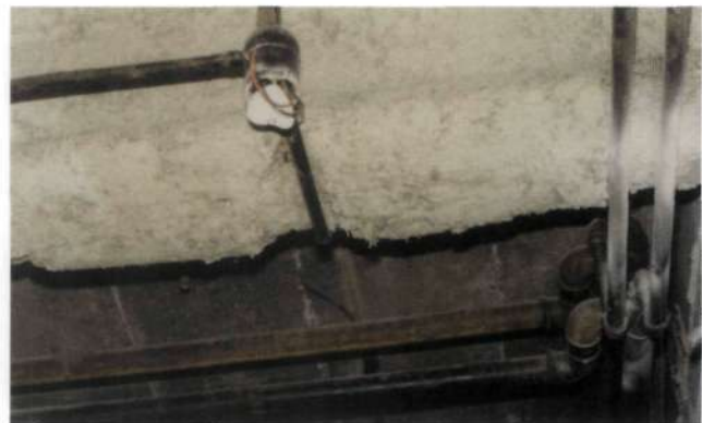
Figure 48b Poorly tamped sprayed chrysotile fireproofing on a structural steel beam holding up a concrete floor, showing some overspray onto the concrete and damage by electrical work
