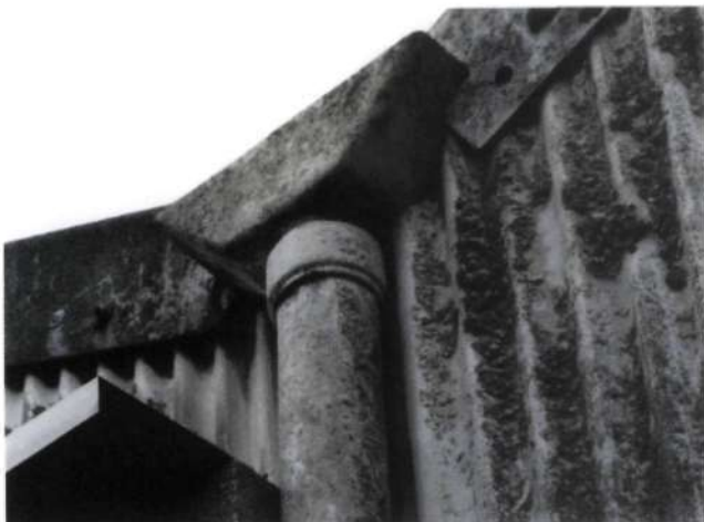
Figure 48d Asbestos cement downpipe, hopper and profile sheet
