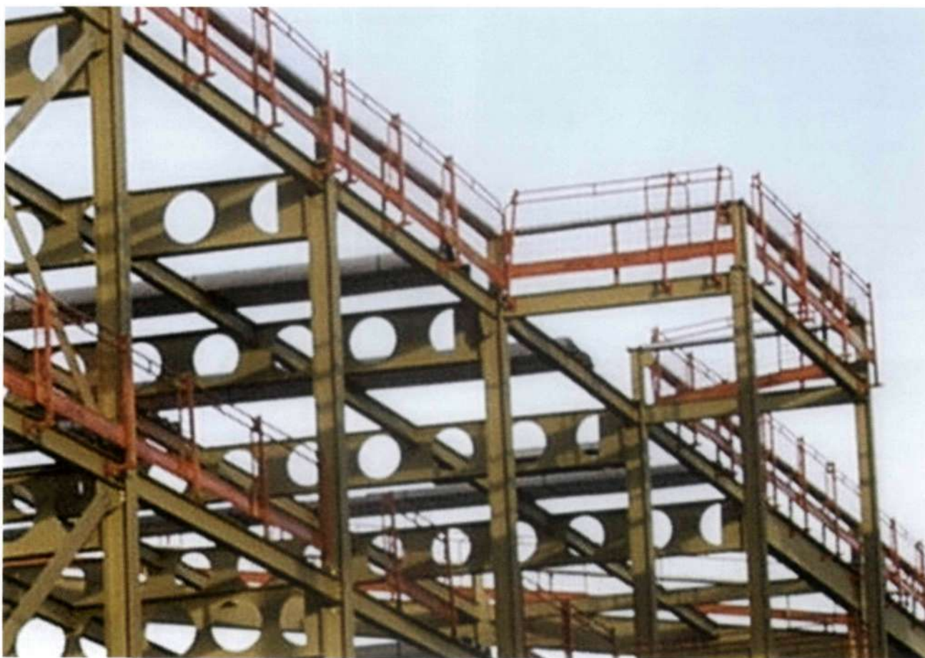
Figure 28 Edge protection installed with the steelwork
