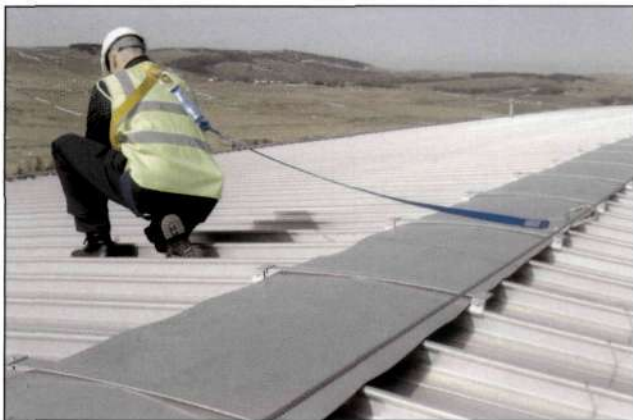
Figure 16 A work-restraint harness
