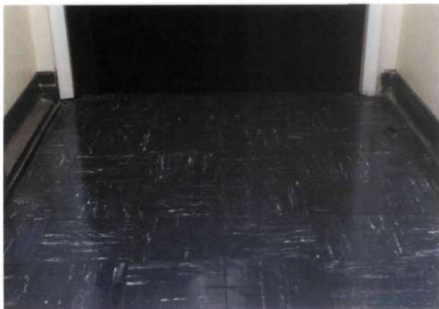
Figure 48e Asbestos-containing vinyl floor tiles
